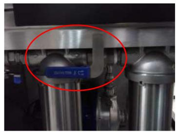
There is also another drain valve situated lower down on the pump (shown here in the "off / normal position). This is used to drain any remaining fluid in the pipework along with the pump drain plug for a complete drain-down of the system:
